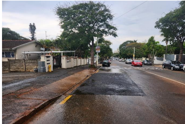
Photos above: Water department repairs of major water leak and reinstatements
