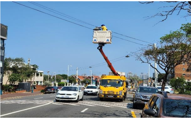
Photo above: Electricity department repairing faulty hanging lights
