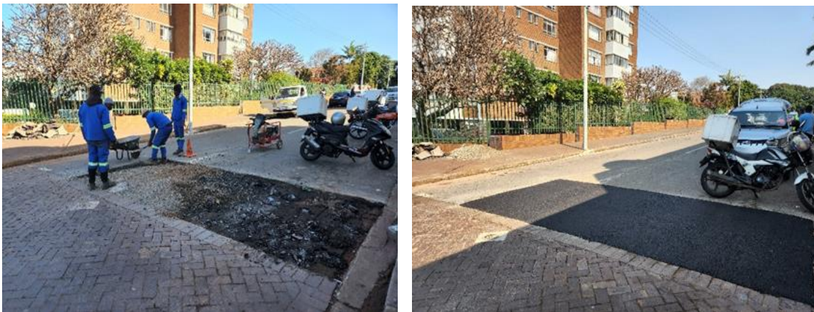
Photos above: Roads department reinstating tar after a waterpipe burst.
