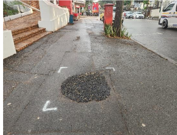
Photos above: Roads department reinstated tar to damaged surfaces.
