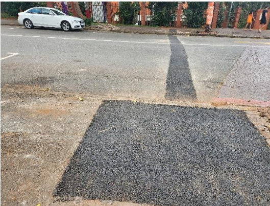
Photos above: Roads department reinstated tar to damaged surfaces.
