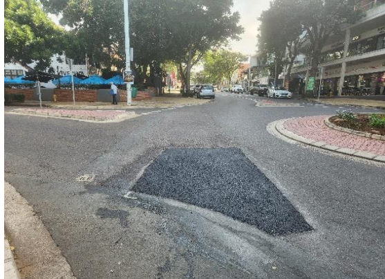
Photos above: Roads department reinstated tar to damaged surfaces.
