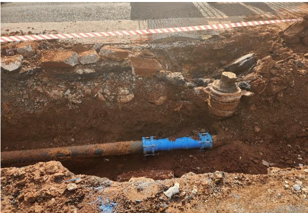
Photos above: Water department repairs of major water leak and reinstatements
