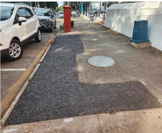
Photos above: Roads department reinstated tar to damaged surfaces.
