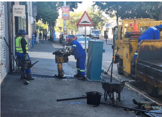
Photo above: Roads department repaired a sinkhole on the sidewalk.
