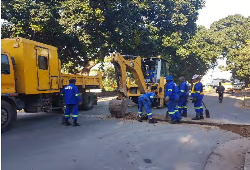
Photo Below: Reinstatement of tar to road surface after power cables were installed
