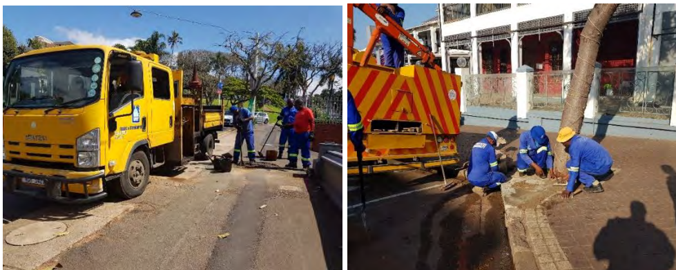
Photos below: Roads Department repairing drainage cover
